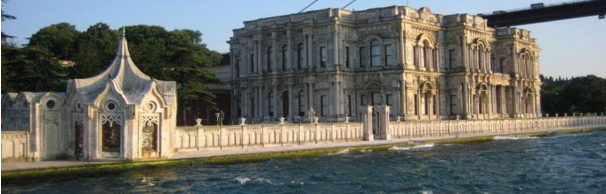
Figure 4. Sea wall and pavilion overlooking the Bosphorus
